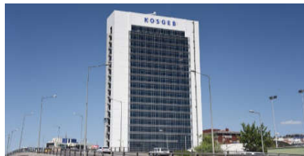
KOSGEB BUILDING (ANKARA)
