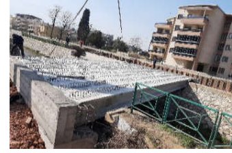
PRESTRESSED BRIDGE (KESTEL)
